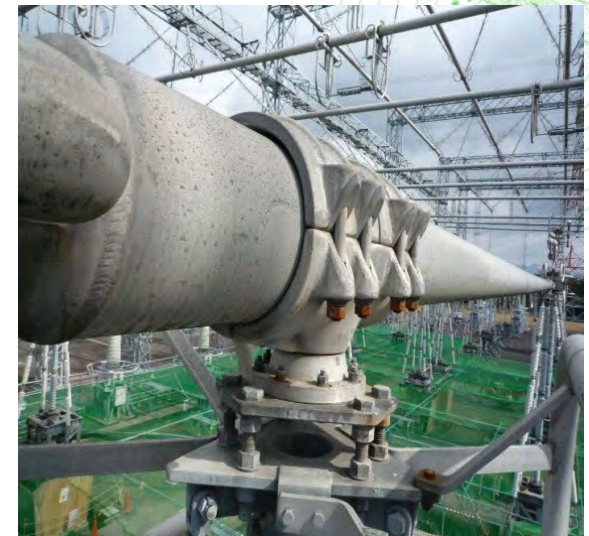
Aluminium bracket with a slide support mechanism
